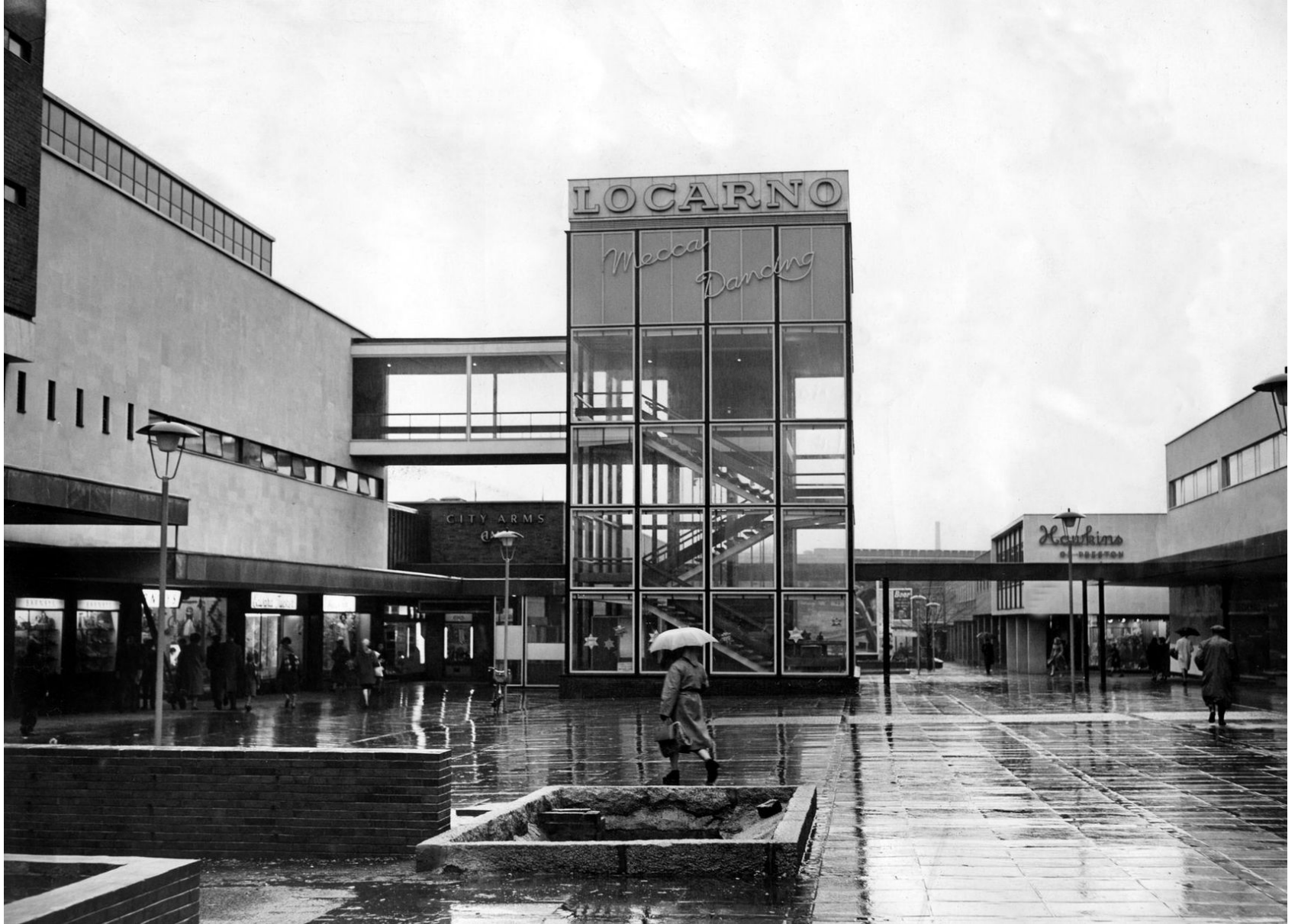
The glass tower entrance to the Locarno club in Smithford Way Precinct, Coventry, in 19603 of 10
